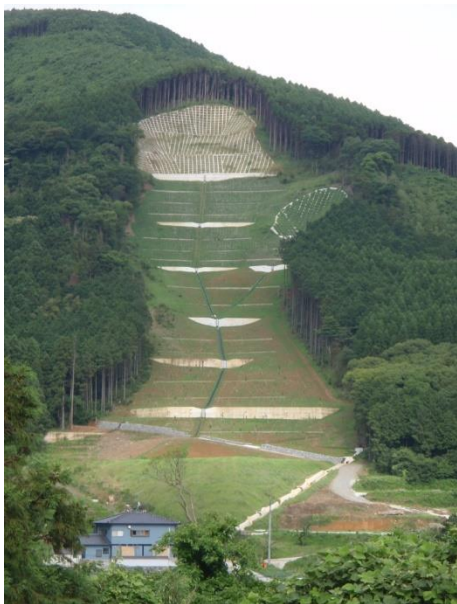
[土留工、法枠工]
