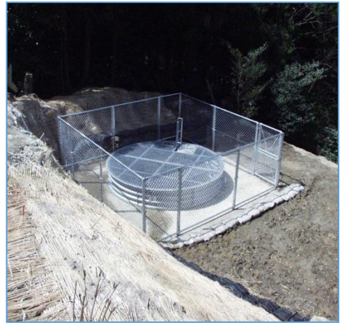
[地すべり防止工（集水井工）]
